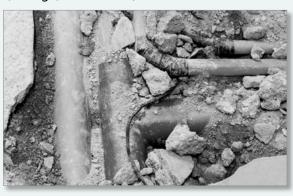
Fixture Supply. A water supply pipe connecting the fixture with the fixture branch.
