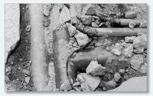
Fixture Supply. A water supply pipe connecting the fixture with the fixture branch.
