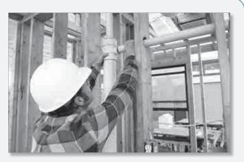
a soil or waste stack or building drain with or without vertical sections or branches, which receives the discharge from one or more fixture drains and conducts it to the soil or waste stack or to the building drain.
